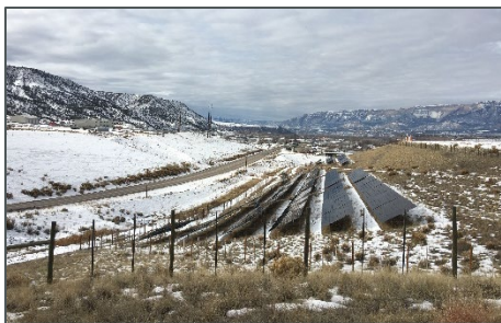
Solar array at Rifle Garfield County Airport
