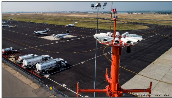
Remote tower project at Northern Colorado Regional Airport (Shahn Sederberg, CDOT)
