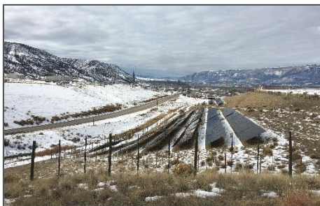
Solar array at Rifle Garfield County Airport
