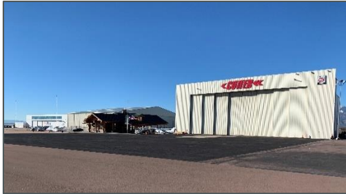
Colorado Springs Municipal Airport
